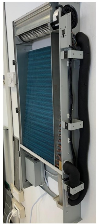
PUT INSULATION IN ALL THE EXTERNAL PIPE
