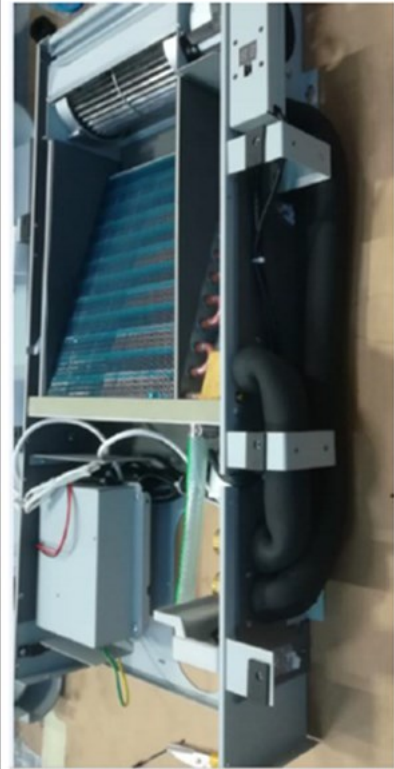
PUT INSULATION IN ALL THE EXTERNAL PIPE
